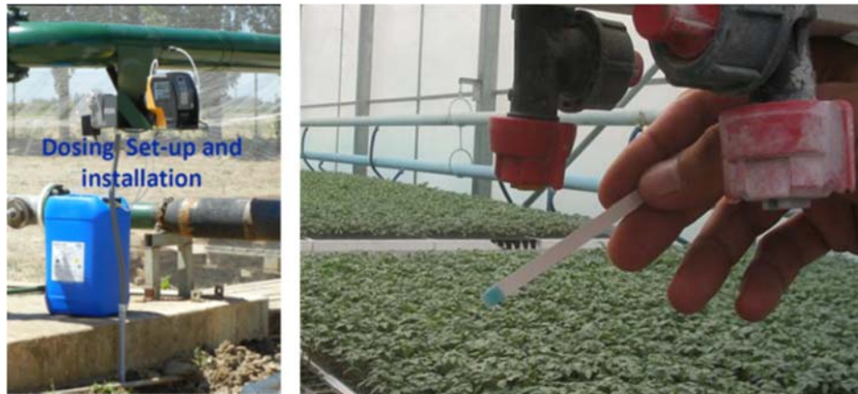
Figure 1. Left: illustration of a dosing system with a pump controlled by a water meter. Concentration: 20-40 ppm. Right: simple measurement at the end of the pipeline by means of a test strip.
